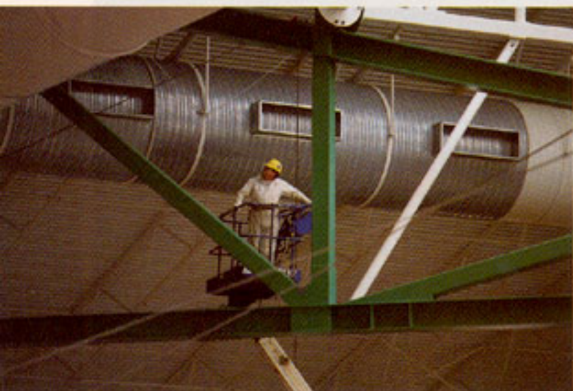
LARGE air-handling ducts will keep indoor environment under control.
