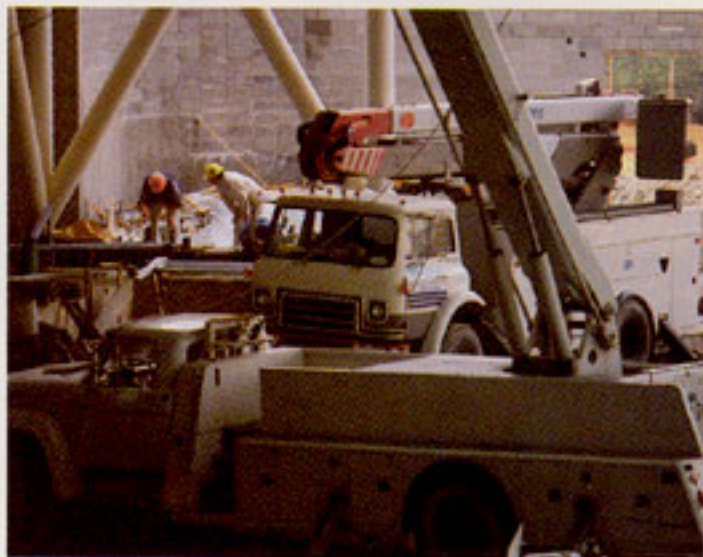
COMPLEX is large enough to accommodate large trucks.
